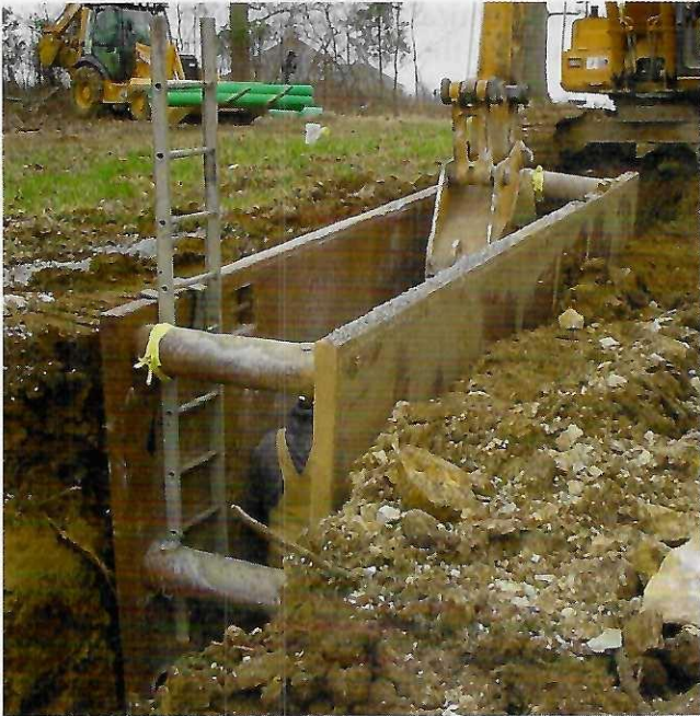
Figure 37 Ladder in a trench.
