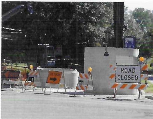
Figure 20 Work zone signs and tags.
