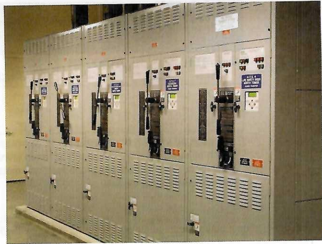
Figure 2 Typical low-voltage, metal-clad switchgear.
