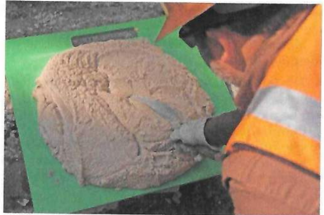
Figure 30 Picking up mortar from a board.
