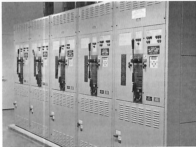
Figure 2 ♦ Typical low-voltage, metal-clad switchgear.
